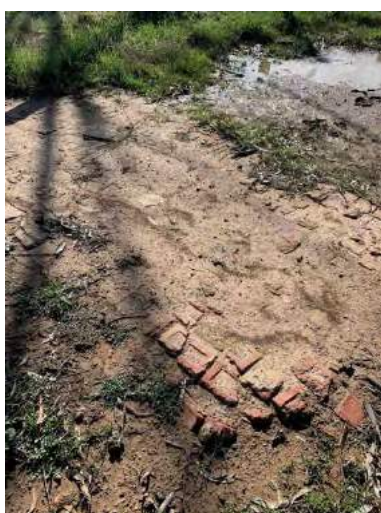
Figure 3-1: Bricks used to build up gateway area
